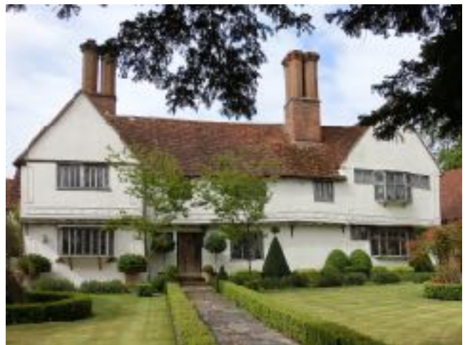
Brook House at North End, Felsted
